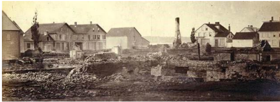
After the fire, looking toward Water Street
