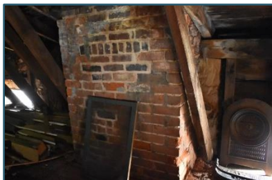
Figure 31: Chimney brick from attic
