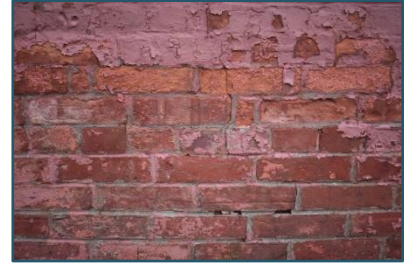
Figure 81: Cracking in foundation on south facade
