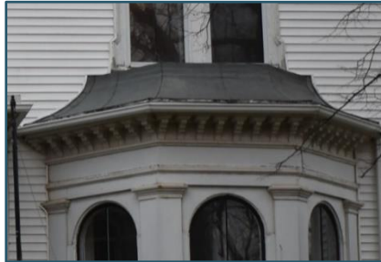
Figure 106: Roof over southmost bay window on front facade
