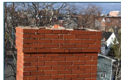
Figure 30: Failed parge
