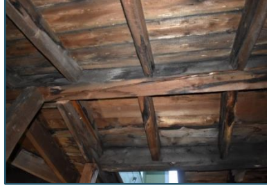
Figure 35: Failing beam
