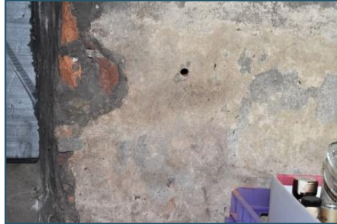
Figure 110: Borescope opening 2
