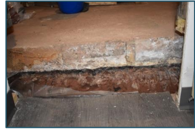
Figure 96: Poured concrete slab
