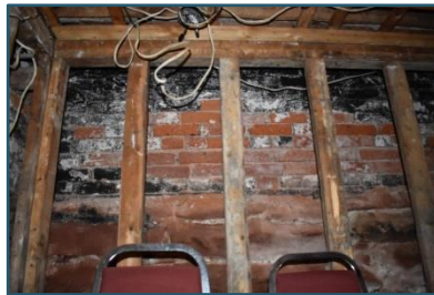
Figure 86: Revealed foundation at front facade
