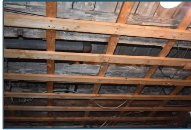
Figure 95: Revealed ceiling framing
