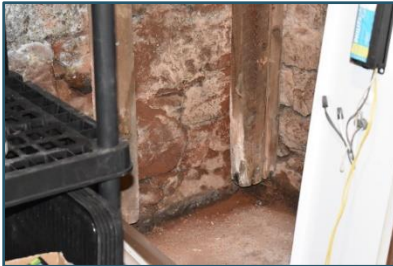
Figure 97: Framing shows where ground was before being lowered
