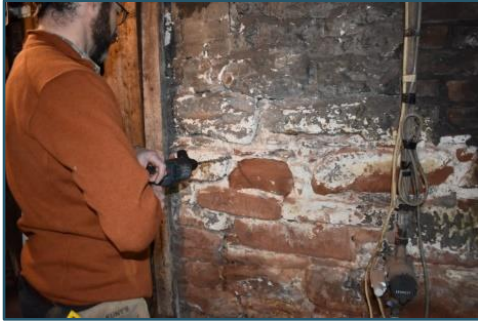
Figure 109: Borescope opening 1
