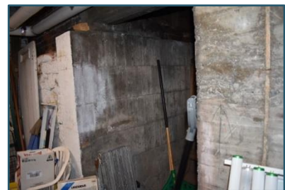
Figure 90: New concrete foundation
