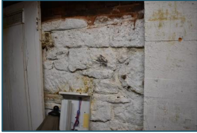
Figure 91: Painted masonry foundation
