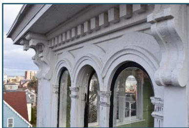
Figure 28: Failing paint
