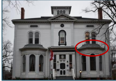
Figure 38: Lower roof on southmost bay window circled in red, viewed from Haviland St.
