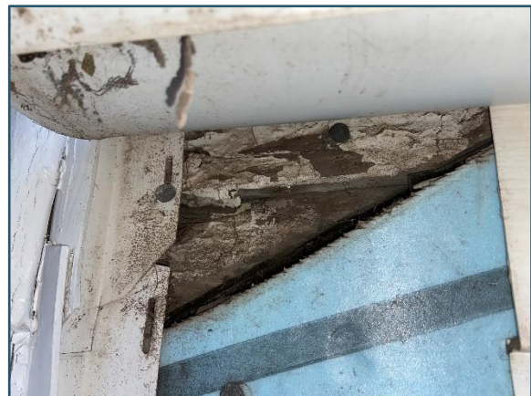
Figure 111: Wood siding under vinyl, photo provided by Greg Munn 2022-12-21
