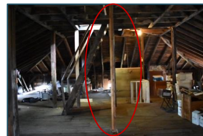
Figure 33: New support post
