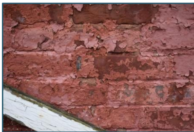
Figure 73: Failed paint
