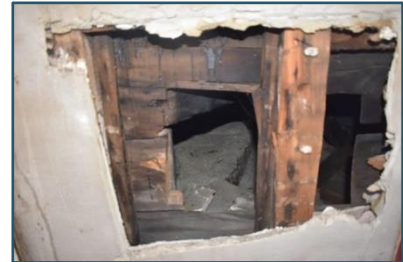
Figure 54: Opening into wall
