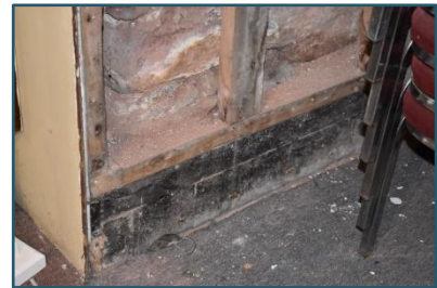
Figure 87: Concrete underpinning on front facade foundation
