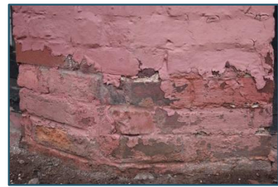
Figure 78: Repair brick and mortar visible
