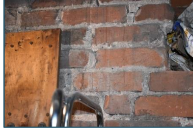
Figure 104: Failing mortar
