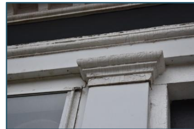
Figure 16: Paint buildup
