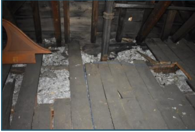
Figure 37: Settled insulation
