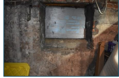
Figure 105: Parging over masonry
