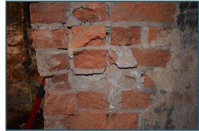
Figure 99: Deteriorated brick
