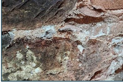
Figure 103: Mortar removed to reveal strong historic mortar underneath
