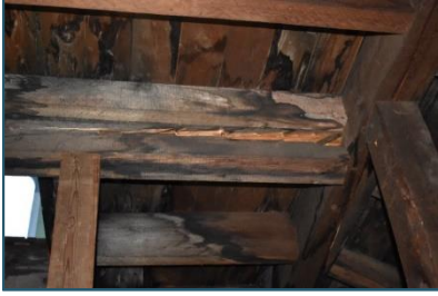
Figure 34: Failed beam
